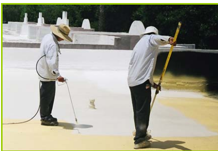
Silicone elastomeric coating being applied
