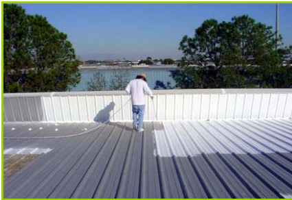
Cool roof coating being applied
