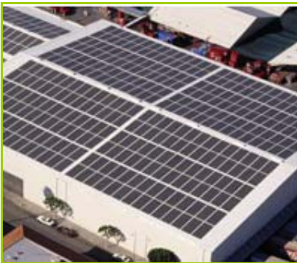
Thin-film BIPV roof system
