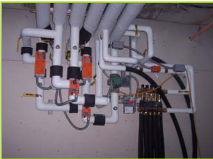
Manifold installation in storage room
