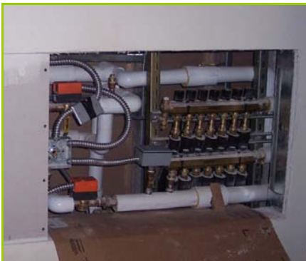
Manifold installation in wall
