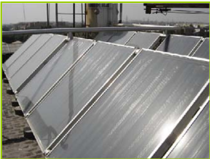
Glazed Flat Plate Collectors
