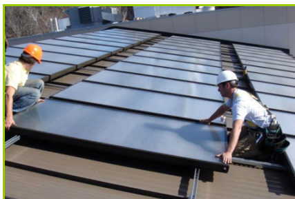
Glazed Flat Plate Collector Installation
