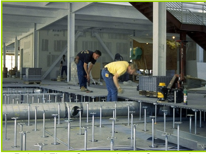
Raised Floor System during Construction
