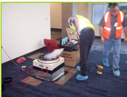
UFAD Commissioning with Smoke to Detect Leakage Paths
